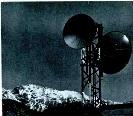
Snow-capped peaks of California form the background for this repeater station. The mountainous area offers the advantage of ready-built tower heights for the line-of-sight requirements of microwave communication.
