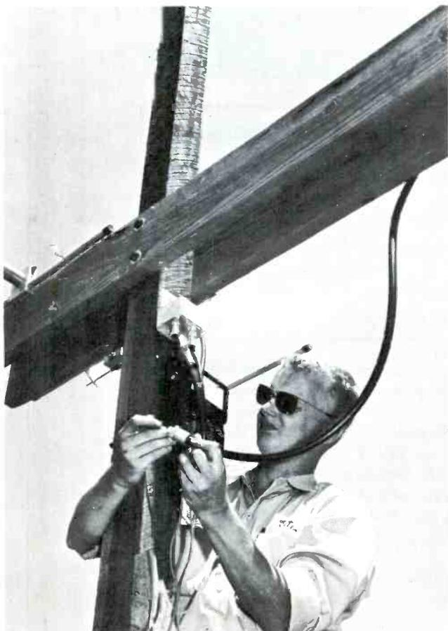
CLOSE-UP OF TECHNICIAN, running continuity test on 1/2 inch 75 ohm Corr-O-Foam cable.
