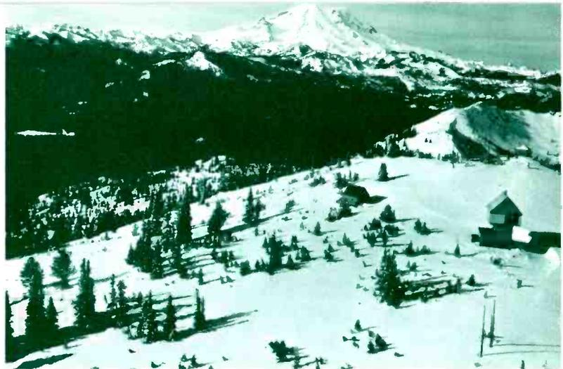
Ravens Roost microwave site in the Cascades at 6,200 feet elevation. Third floor of the building houses the microwave antennas.
