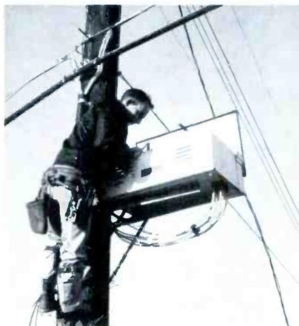
Davco field engineer Tommy Kinion applies finishing touches to rebuilt and re-installed Entron trunk amplifier.
