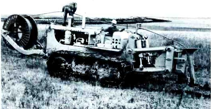
Commercially-built units, such as the ATECO plow shown here, require small crew; provide "plus" features such as steerable plow and hydraulic loading spool carrier.
