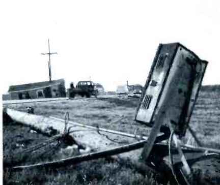
No communications pole lines remained intact—all CATV amplifiers were submerged.
