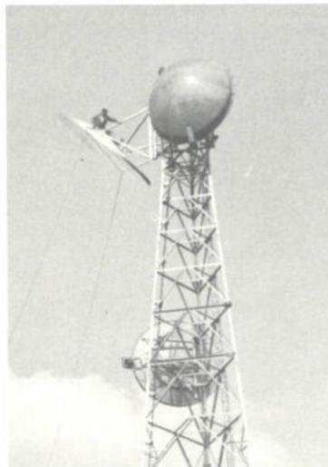
Elliptical tower-mounted reflector being installed atop self supporting tower.
