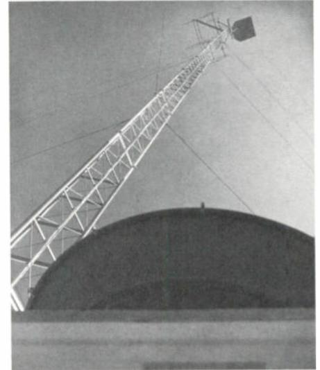
Figure 3. VHF arrays atop Chatsworth, N.J. tower receive New York channels for relaying via microwave to Milmay.
