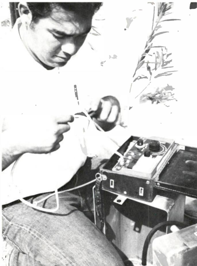
*Installer Sebastian Ponce is shown running field test at pedestal location. Advantage over pole- or strand-mounted equipment is obvious in maintenance work.*
