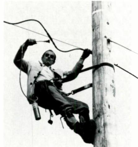
Here San Jose Cable TV technician Joe Hepburn makes a heat-shrinkable splice cover on an overhead coax. Propane torch adds little weight to climbing gear.
