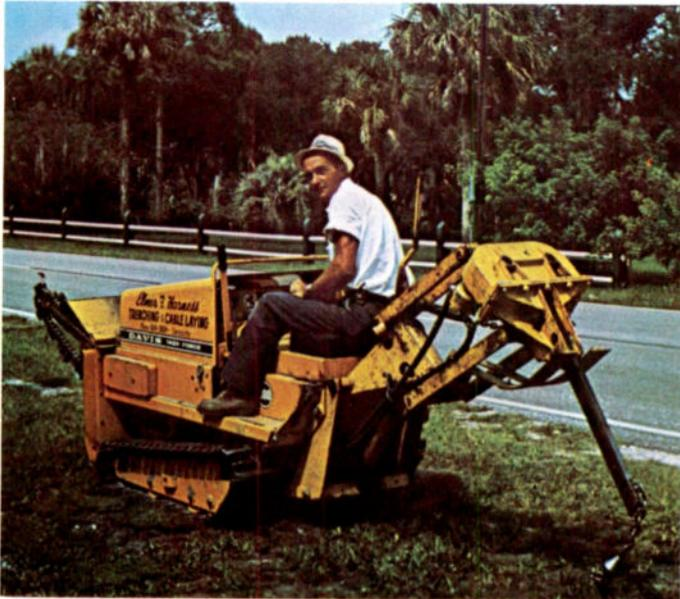
Use of a vibratory plow for direct burial of trunk and feeder lines is big improvement over trenching.
