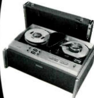
The "VTR" output of the TMV-600 can be switched to either preview or program switcher buss, permitting recording sessions without disturbing "on-air" operation. Video outputs of each VTR connect to separate switcher inputs.
