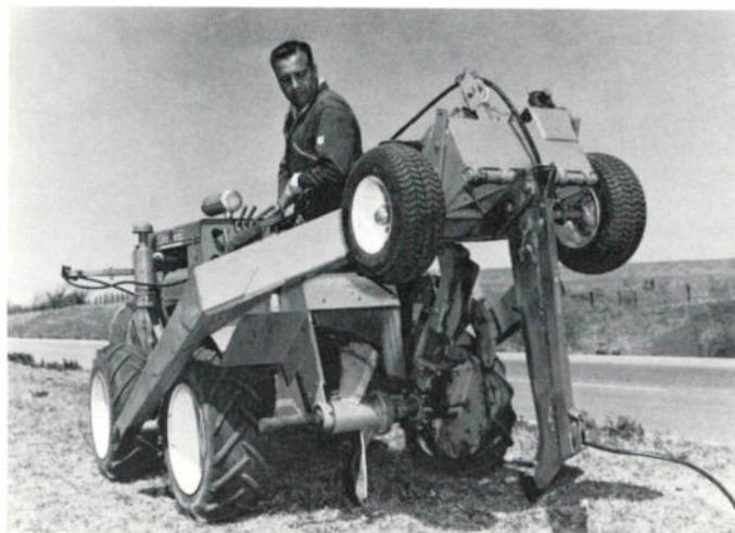
Optional plow attachment quickly converts 30-horsepower trencher to vibratory plow for direct burial of cable. This trencher model provides trenches of up to 18 inches wide, 6 feet deep, and is equipped with hydraulic backfill blade. Additional attachments convert basic trencher into backhoe or boring unit. Will handle all sizes of distribution cable.
