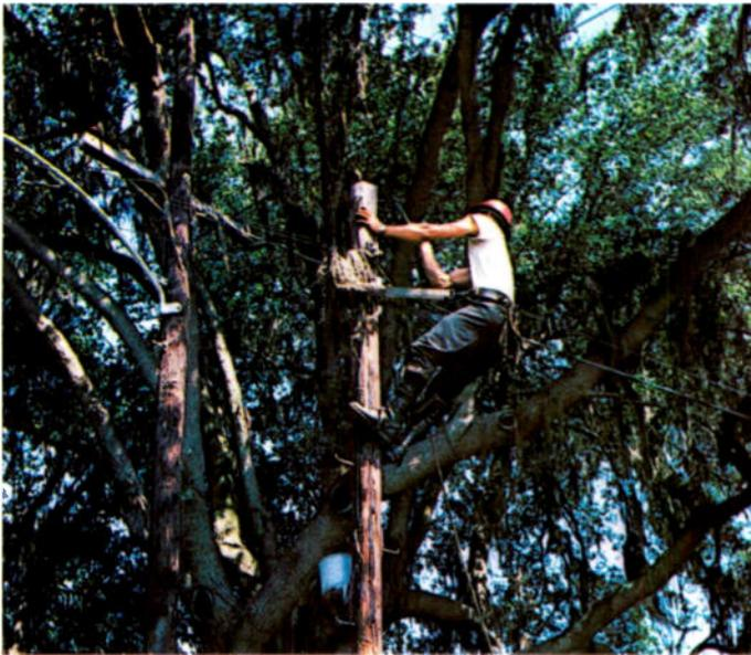
*City-owned utility poles are used in the Lakeland plant — stranding crews kept cables 12 inches below telephone lines, 52 inches below power lines.*
