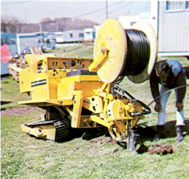
*Start of direct burial run, with vibratory plow in ground, is shown here. The method eliminates trenching, hand laying of cable, and backfilling.*
