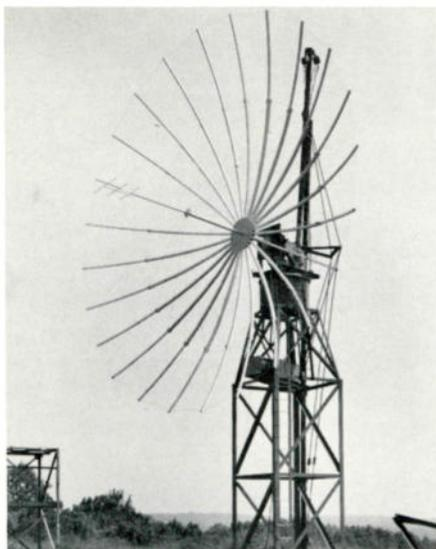
**30 Ft. Parabolic Antenna.** All channels from a given area can be received with one antenna and one feed. By positioning feed in parabola, a null can be placed in direction of undesired channel. Covers all UHF and VHF channels; steel and aluminum construction.
