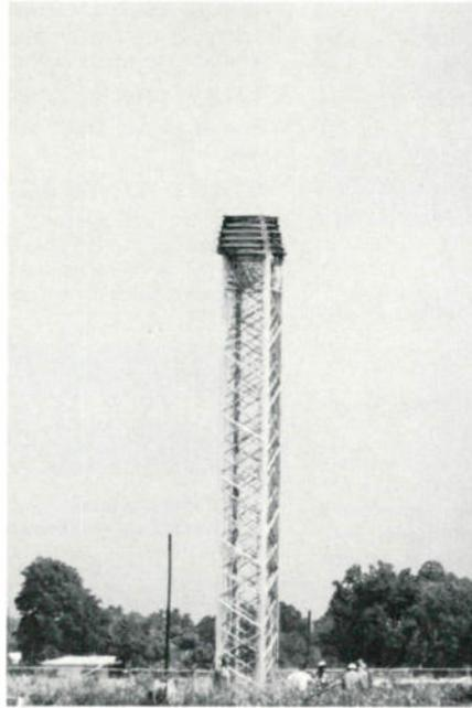
Stacked sections are pulled upright by tower guy wire. Rising sections pull remaining guys into place. No extra equipment required.
