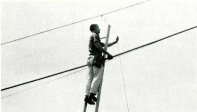
Recently installed drop cable has been conveniently draped across telephone line, apparently to avoid the expense of setting a pole or making a buried street crossing.
