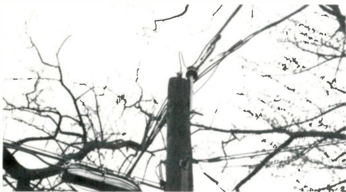
Above: Cable on top of this pole is just 3 inches from 220 v. power conductor. Even attached at top of pole, the cable is 4 ft. below minimum clearance over adjacent street. However, the cable was attached at the 15 ft. level on pole across the street, and could have been elevated 4'6" without rearrangements.
