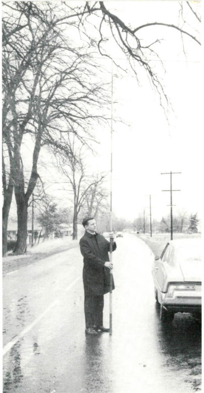
Above: Fiberglass measuring pole is used by TVC publisher Stan Searle to check clearance over street. Drop cable is 14'1" over traveled portion of roadway, nearly 4 ft. below minimum.
