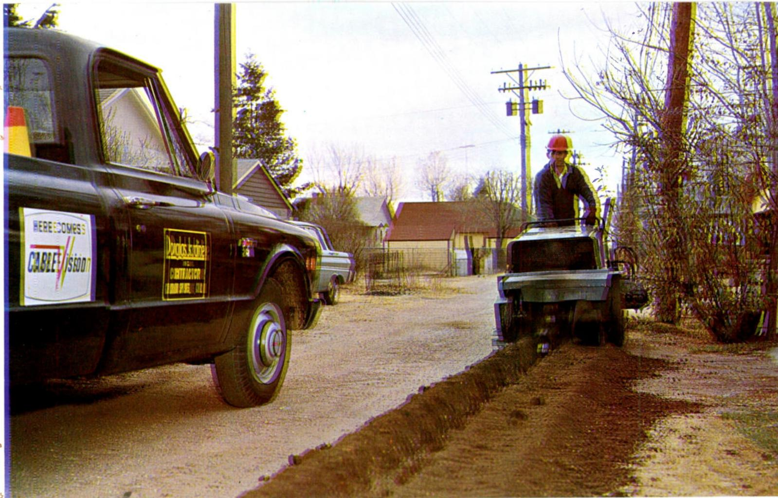
Over 400 miles on underground plant make up the Colorado Springs system. The Davis trencher shown is cutting a trench 5" x 24".
