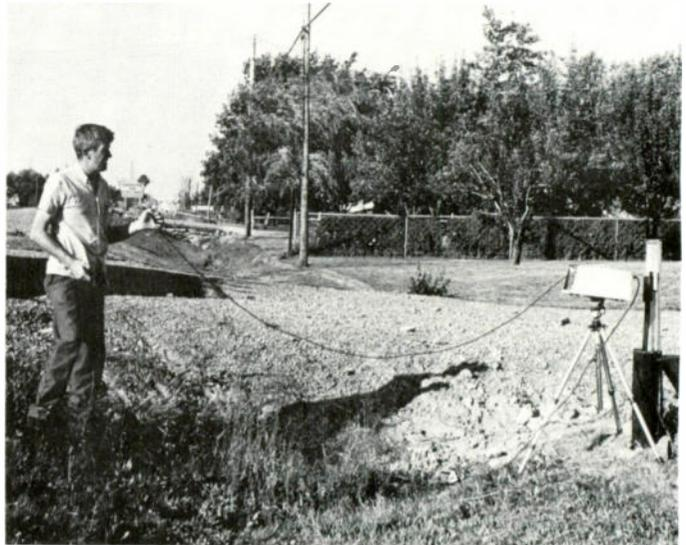
After preparing film and X-Ray unit, the technician steps well back and uses remote control cord to actuate X-Ray mechanism.
