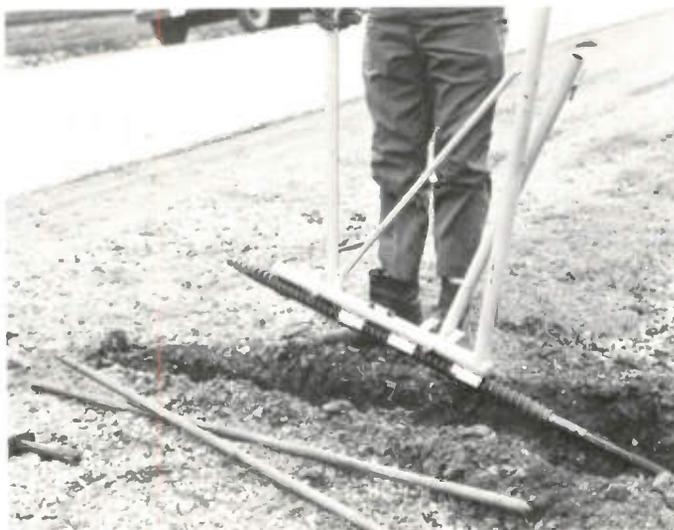
Here the boring head is cradled in the guide tool, ready for positioning in starting trench.
