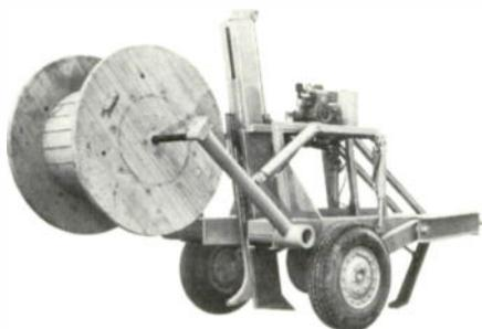
safety relief spring, plow tooth vertical adjustment from 0° to 50° and front jack stand. Plow tooth thickness from 2" to 4" is available and the unit buries material up to 3½" O.D. or larger with modifications.
