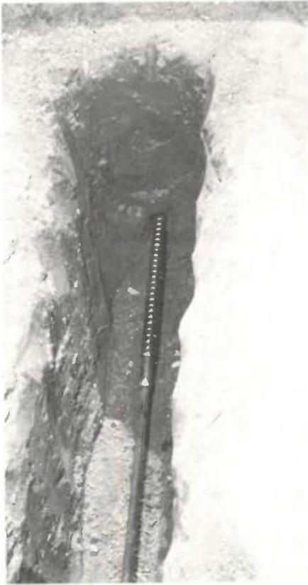
The boring head has been started in the soil. The guide tool, has been removed to show detail.
