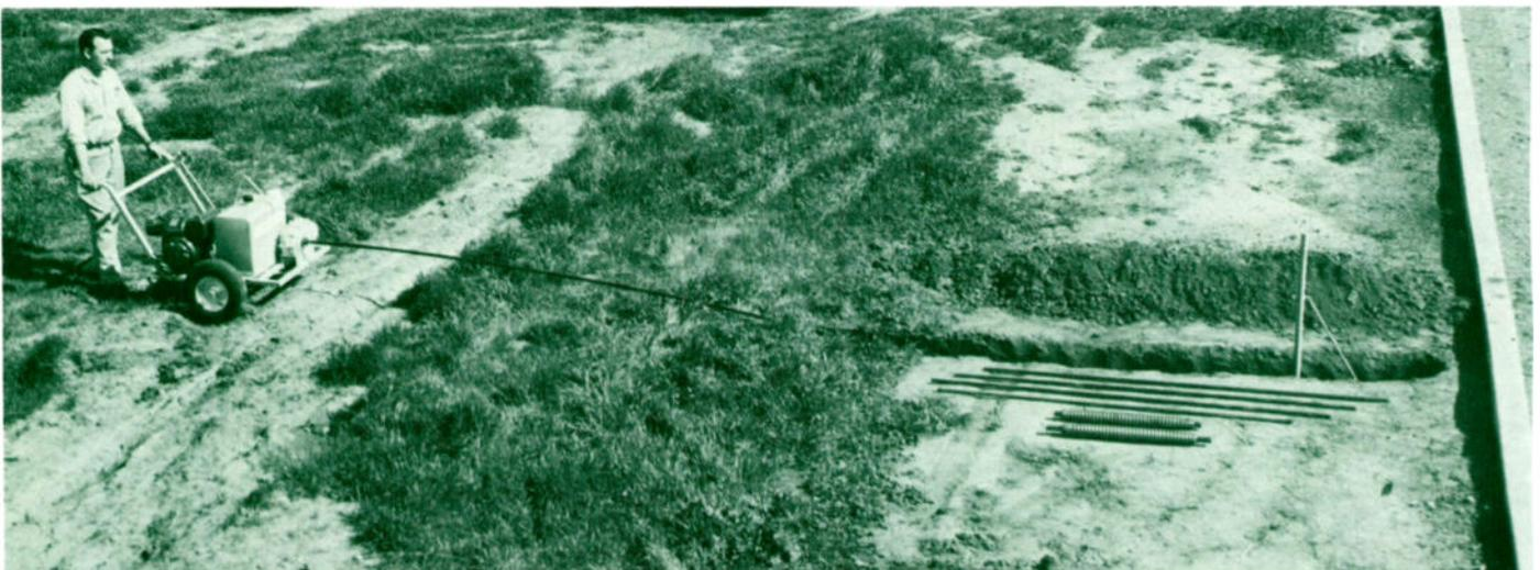
The compacting auger operation is shown in progress here. After the bore is completed, coaxial cable or conduit can be installed by swivel attached to reamer on return pass, or cable can be hand fed through the bore.
