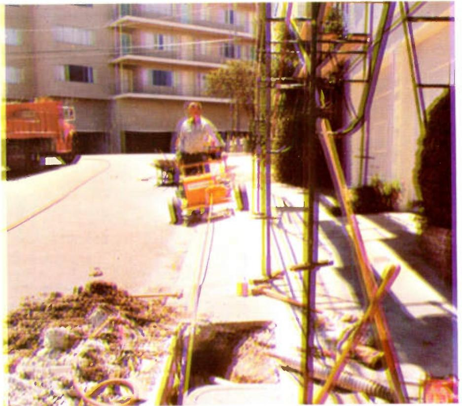
The Undertaker compacting auger has been used in the Twin Peaks area of San Francisco to install coaxial cable under sidewalks. As illustrated above, dry-bore operation does not require large access openings.
