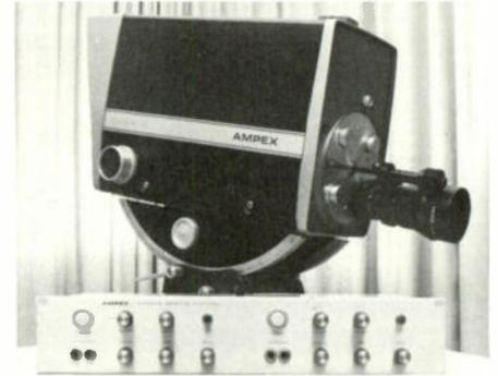
unit operator. Two headset receptacles on the camera and on the remote control accept standard telephone operator headsets. The CC-327 camera sells for \$2,700. Single camera control unit is \$300 and double camera unit is \$550. A 25-foot length of cable with connectors is \$250.
