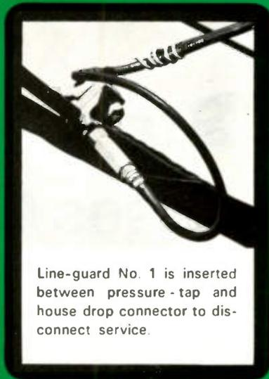
Line-guard No. 1 is inserted between pressure-tap and house drop connector to disconnect service.
