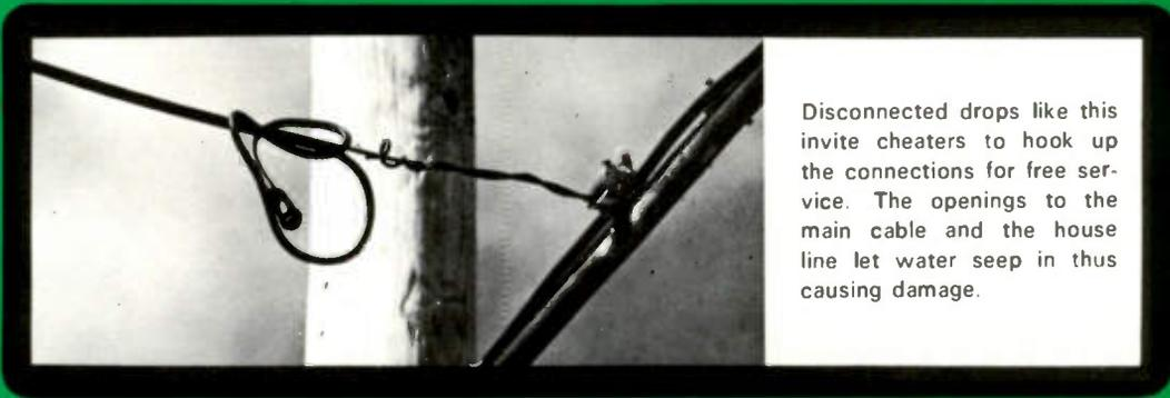
Disconnected drops like this invite cheaters to hook up the connections for free service. The openings to the main cable and the house line let water seep in thus causing damage.
