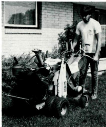
No other machine of its kind can equal PIPE PIPER for speed, maneuverability, and low labor cost. You can bury wire, cable, or flexible pipe around corners and obstacles in one continuous operation. There is no damage to the finest turf and no trench to fill. Constant burying depths of from 5 to 14 inches are easily maintained with one setting. PIPE PIPER is easily transported in a van or trailer.
