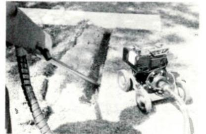
Drills under sidewalks in 5 seconds using our special side-walk auger and extension with wiggle joint.
