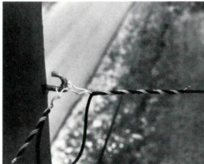
Service wire is safely and neatly brought into house with two TELEGRIPS. Unique helical construction cradles cable to prevent "snowy" distorted picture.
