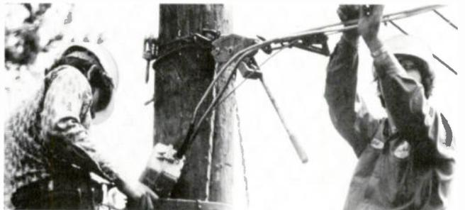
Messenger which supports feeder cable is tensioned with come-along prior to permanent attachment to pole fitting with PREFORMED GUY-GRIP® Dead-end.
