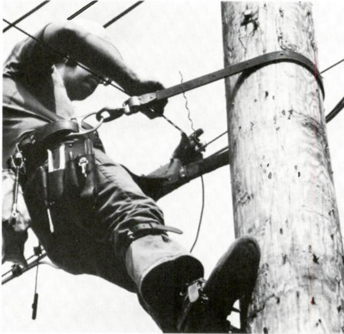
Construction crewman needs only seconds to apply PREFORMED Custom Coaxial Dead-end while making a pole transfer. One piece construction is quickly applied by hand without tools.
