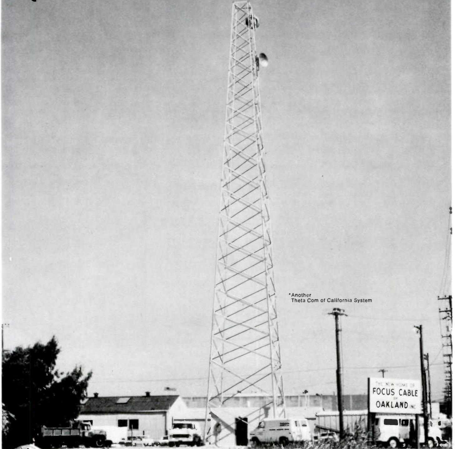
The Tri-Ex SQUARE RIGGER TKD-4-120. Self supporting. Rock-solid steady on four legs. For microwave installations.
