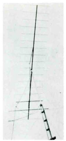
Hosken's 17 element low band (2-6) yagi. 15 db. gain.
