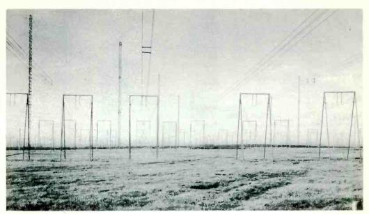
Antennas—antennas everywhere...as far as the eye can see. A "portion" of the BBC General Overseas Service Antenna System, seemingly stretching to the horizon. The four wire feeder systems are supported by the smaller towers. The larger towers support the actual antennas, "Sterba Curtains" mostly.
