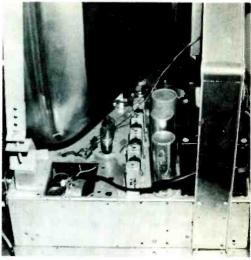
"Mattison receiver in service at DXH. The tuner is submounted in the well, front left. Five 1.F. cans and four IF tubes run in a straight line off center to the right, and at far right, the transformer power supply."
