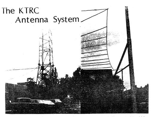
One of the more interesting tower installations is at KTRC, Santa Fe, New Mexico, which operates on 1h00 KHz with 1 kW fulltime. They faced a problem that a number of AM stations have had to deal with- the real estate where their ground system is plowed into the ground becomes almost as valuable as the radic station itself.
