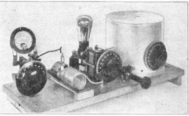
THE LOW-POWER OSCILLATOR-AMPLIFIER TRANSMITTER The oscillator is inside the inverted aluminum kettle at the right with the neutralized amplifier and antenna-coupling circuit to its left. This unit may be used to excite a high-power amplifier.
