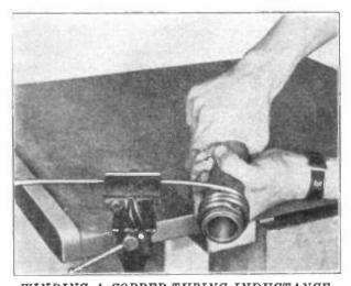
WINDING A COPPER-TUBING INDUCTANCE One end of the tubing is held in the vise and the other is flattened out and bolted to the pipe used as a winding form. Pulling on the tubing and turning the pipe in the hands, the operator walks towards the vise. The turns should be wound as closely together as possible and spaced later.
