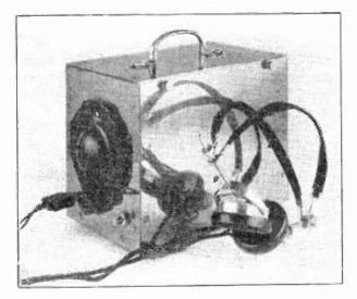
A MONITOR WHICH IS WELL SUITED TO CALI-BRATION FOR FAIRLY ACCURATE WORK It is not, however, as good as the frequency meter described later in the chapter for precise measurement of frequency.
