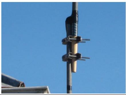
With the u/v bolts, washers and nuts the pipe and rod were joined together. Thanks to Jim Searle.
