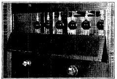
SIX MERCURY-VAPOR TYPE TUBES ARE USED IN THE 550-KW, RECTIFIER
