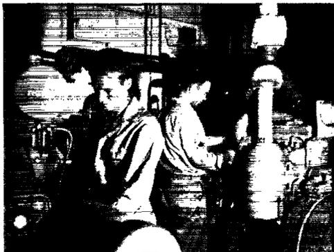
T/Sgt. Harold Hendricks (right), chief power maintenance man, adjusts one of the two three-phase diesel-engine generators, while Cpl. Wm. Hardin inspects the relief generator. Either one or both power units may be used simultaneously to provide as much as 100 kw. for the transmitting gear aboard the *Apache*.
