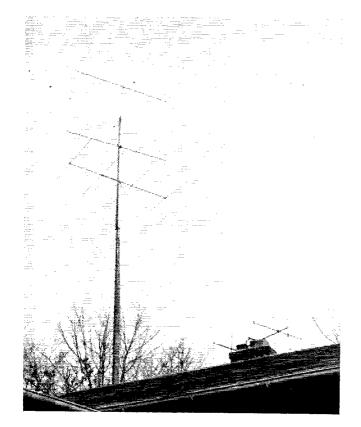
Antennas at W2TBD, Medford, N. J., include a 12-over-12 for 114 Mc, and a 4-element for 50. The 2-meter array is hinged at the center for flop-over operation. Spacing between bays is 1½ wavelengths. The vertical array on the chimney is for the RTTY net.
