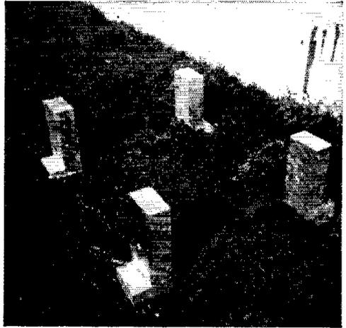
"The exposed ends of the ground posts are notched out to fit the legs . . ."
