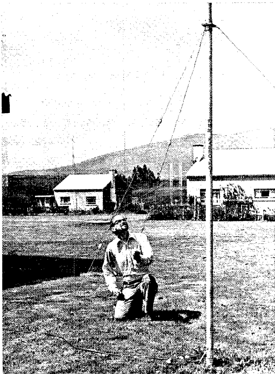
K4ERO/HC1 checks the guys on his 10/15/20-meter vertical.
