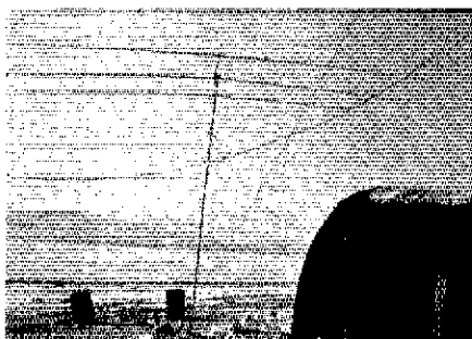
At their base camp at Hazen Lake, K2BPP, N4ZG and K0BJ practiced putting together their 20-meter, 3-element, Hy-Gain antenna. The group was able to install the antenna at the Arctic site in about 15 minutes, a feat made possible in spite of the sub-zero temperatures, because the antenna sections were color-coded. (photo by Dave Porter, K2BPP)
