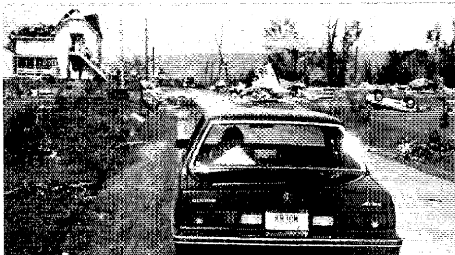
KB3OM surveys the damage in Lycoming County, Pennsylvania. (K3QDA photo)
