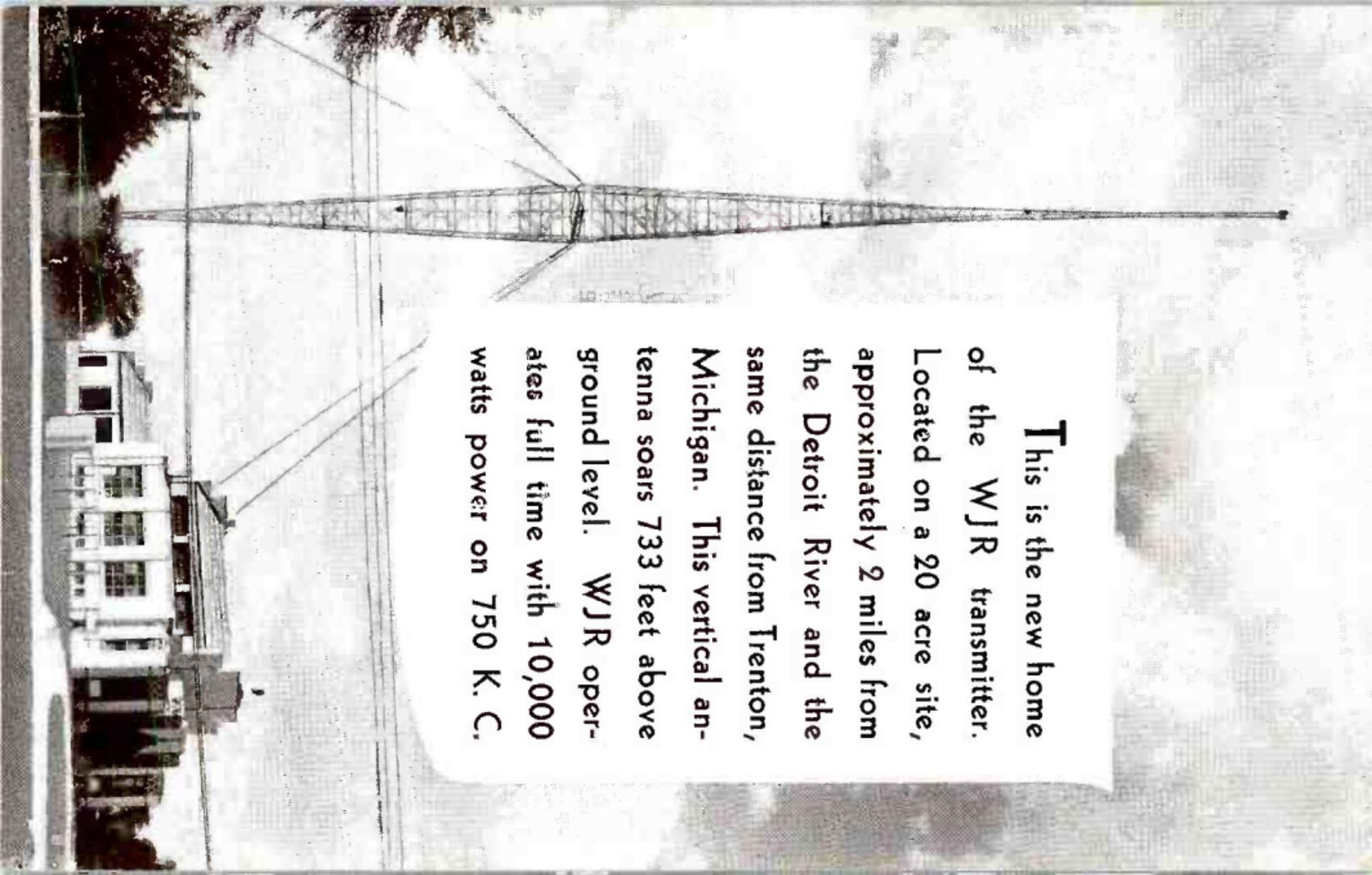
**This is the new home of the WJR transmitter. Located on a 20 acre site, approximately 2 miles from the Detroit River and the same distance from Trenton, Michigan. This vertical antenna soars 733 feet above ground level. WJR operates full time with 10,000 watts power on 750 K. C.**
