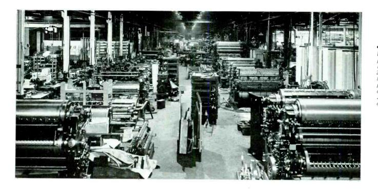
World's largest Offset press plant. This sectional view at H-S-P presents a series of 2-color Offset presses in the long process of careful completion. Producing all forms of color lithography for America's advertisers requires mechanical perfection of equipment.
