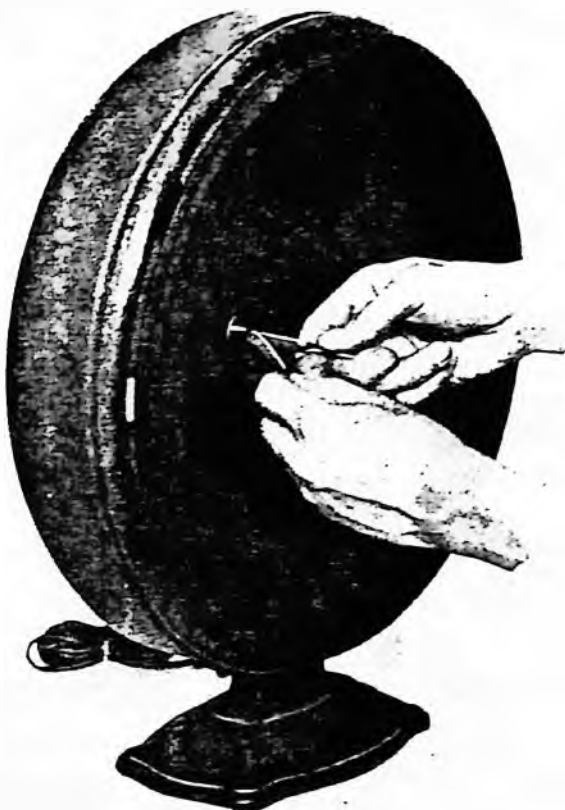
FIG. 86. REMOVING CONE, MODELS E AND E-2.
