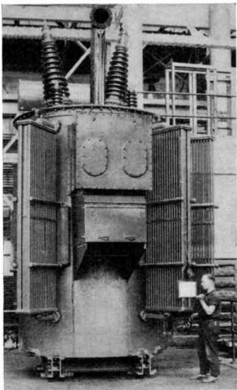
Fig. 1. External View of a Load Ratio Control Transformer
