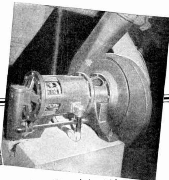
A very high-speed, d-c. motor application—a G-E, 40-hp., 3600-r.p.m. motor driving a G-E centrifugal exhauster in the Halio Bros. Department Store, Cleveland Ohio.
