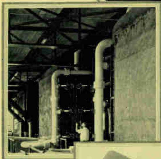
General view of the Foster Economizers installed at the Inglis plant. Characteristic features are—low maintenance, high efficiency, compactness with accessibility.
