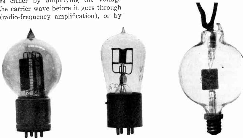
Fig. 9. Three of the Three-element Tubes Used by the Signal Corps of the U. S. Army During the War
