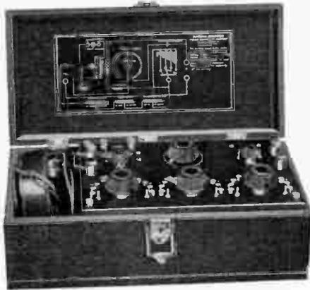
A capacity bridge so calibrated as to be direct reading in capacity. The meter is supplied with a range which makes it suitable for checking the fixed condenser sizes in common use, meeting the need of both manufacturers and service laboratories.
