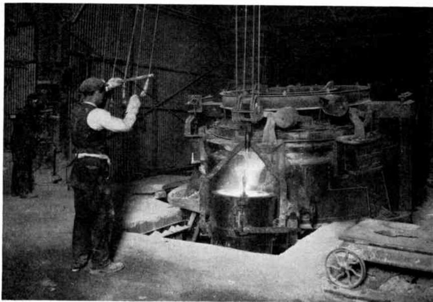
Fig. 67. An Installation of a Horizontal Ring Induction Furnace of 4000-lb. Capacity. The electrical rating is 250 kw., 2200 volts, 15 cycles
