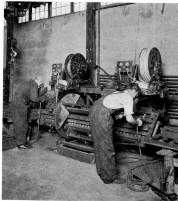
The Apparatus by Means of which Ties Are Quickly Produced from Scrap Rails by the Simultaneous Application of Automatic and Hand Welding Operations
