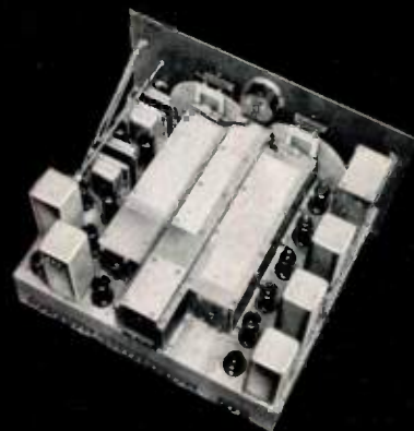
STANDARD 'SUPER-PRO' RECEIVER CHASSIS
