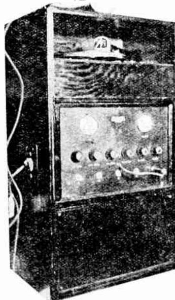
M & H Class "B" Type RD102A Amplifier, complete with tubes, dynamotor, "A" battery and microphone—
