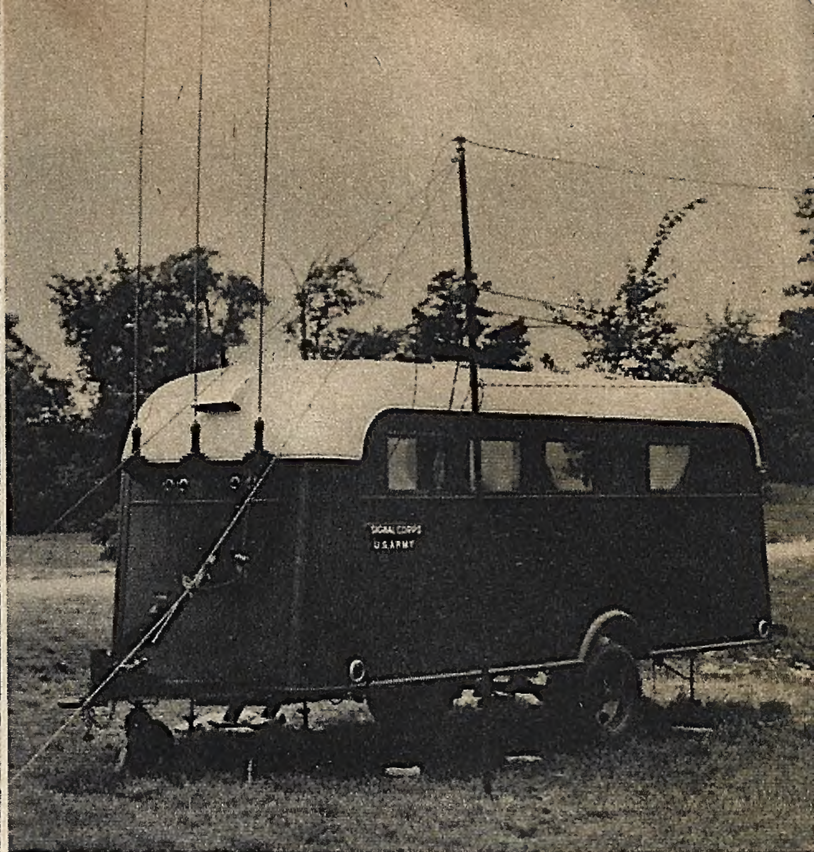
Above, left: Easily concealed, quickly set up or taken down, this loop-aerial equipped radio receiver and transmitter is a favorite in the Army for medium distance communication. Above, right: This trailer is a veritable communications office on wheels. It contains four all-wave receivers and four teletype machines, generates all its own power, is gas-proof, and has special black-out window. Below, right: Inside view of the trailer, showing the receiving position.
