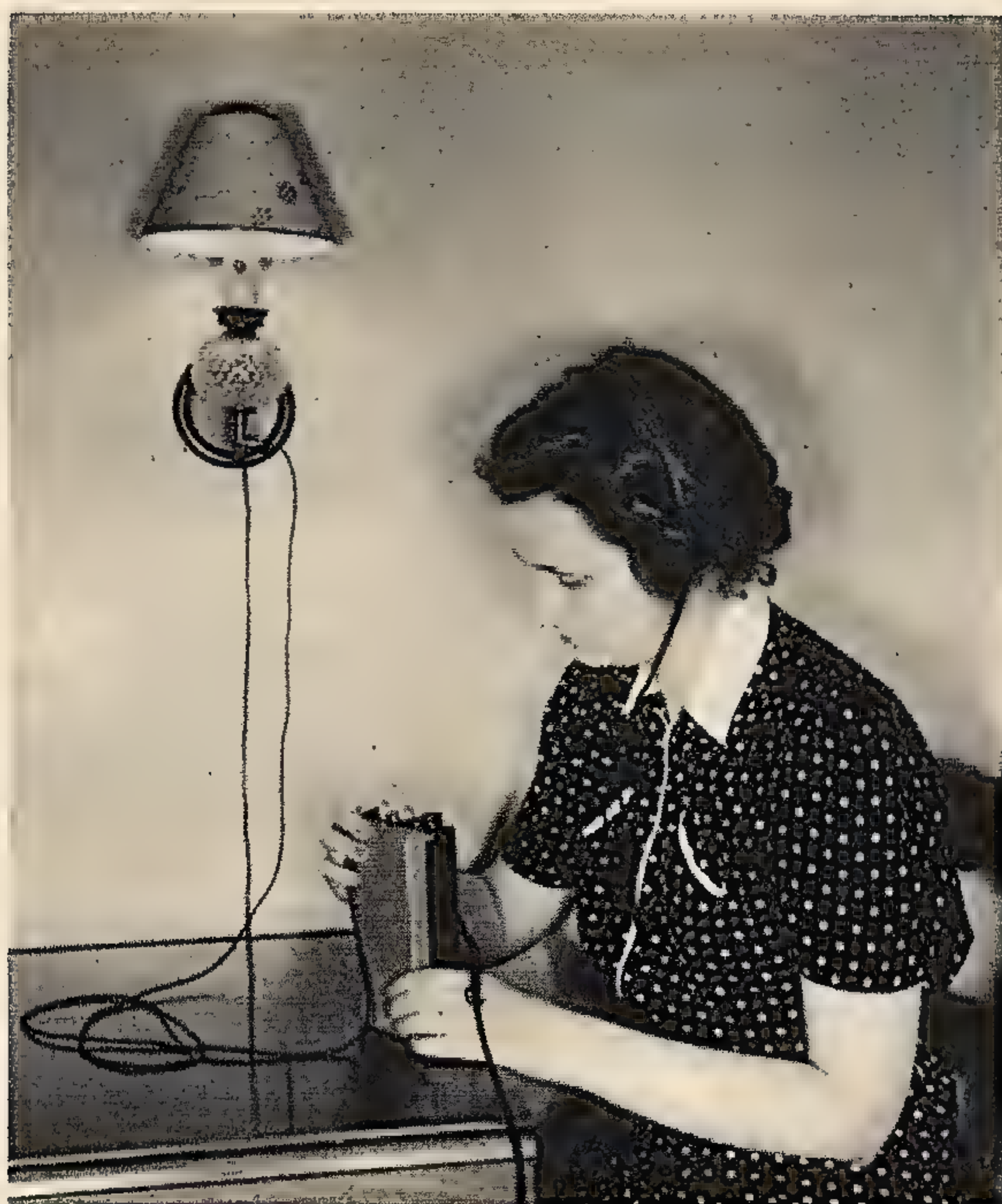
A piece of flexible wire clipped to the electric fixture makes an effective aerial for "Pocket Pete."
