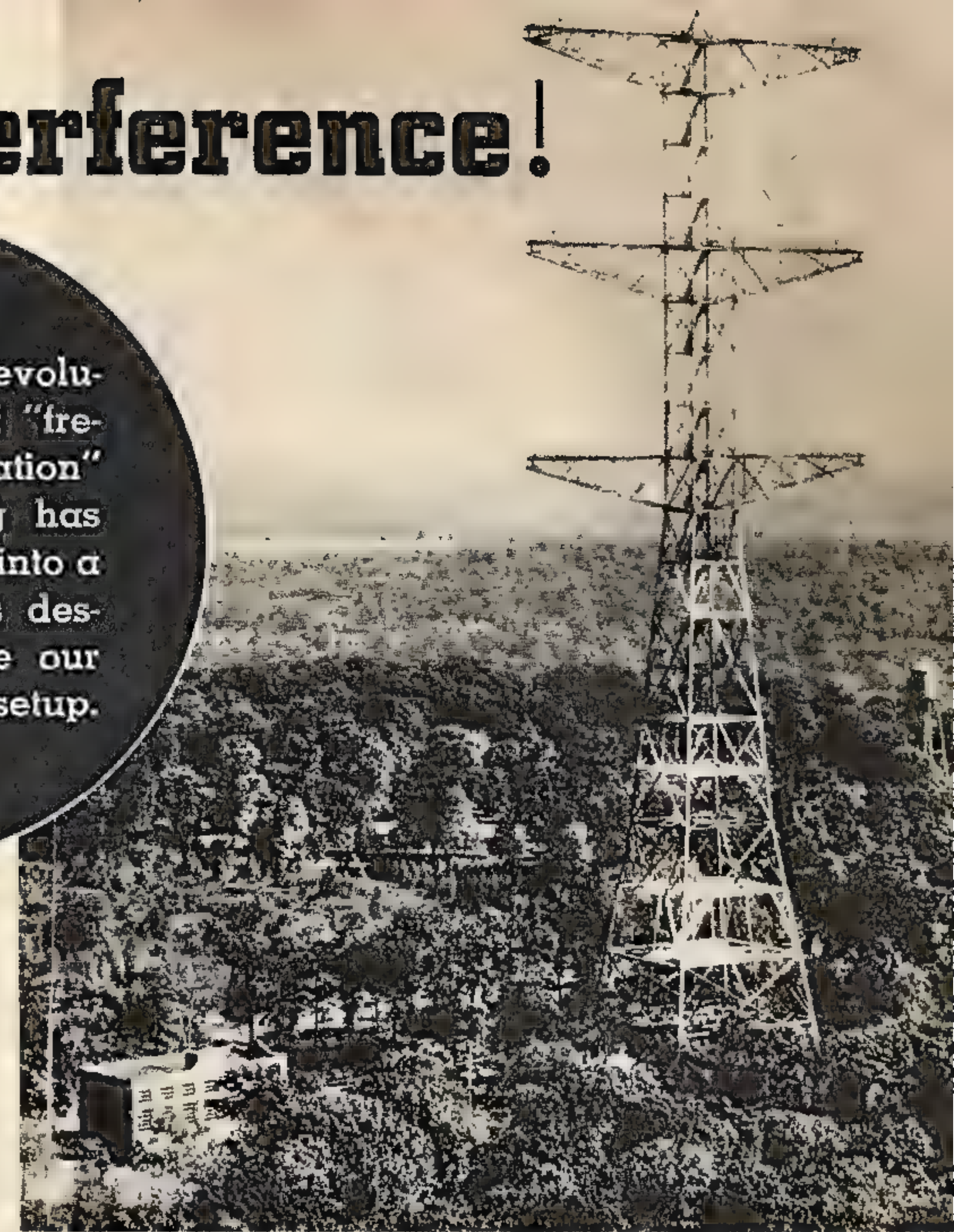
This queer-looking rig is the "turnstile" antenna of Armstrong's station W2XMN, at Alpine, N. J., pioneer frequency-modulation transmitter. It is located on the edge of the Hudson River, just across from New York City.
