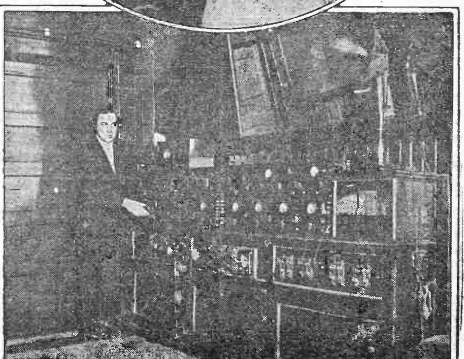
This special super-heterodyne receiver employs twenty-three vacuum tubes and cost more than $3,000
