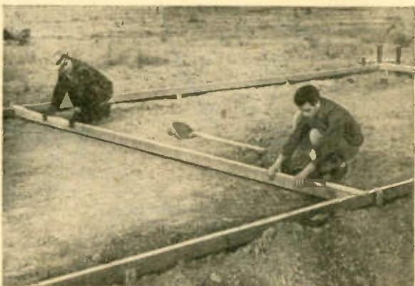
make a final check on squareness by measuring diagonally between line crossings.
