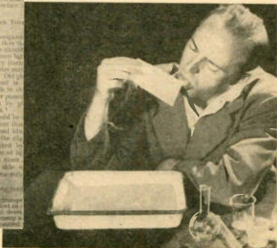
good prints. Too light an image may be due to underexposure in the camera, or underdevelopment in the darkroom. A negative of this kind can sometimes be salvaged by *intensification*. Too dark a negative can be improved by *reduction*.
