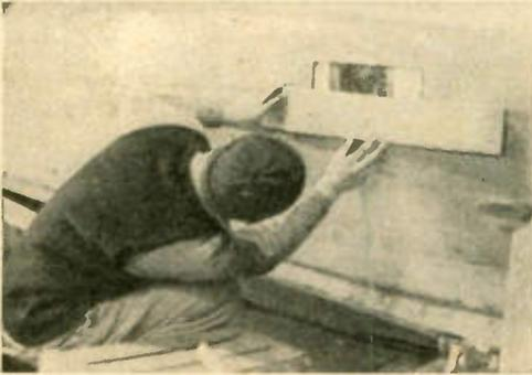
**7** Then a new section of planking is marked up to fit the lower part of the gap. The stock used should be  $\frac{1}{8}$ " thicker than the original on the boat so it can be planed down flush.
