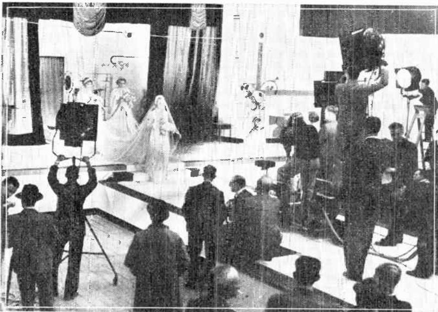
This illustration of a relay of a Mannequin Parade shows the studio technique when the "Electric Eye" is employed. The "camera" is in the centre foreground, and the operator is wearing headphones.
