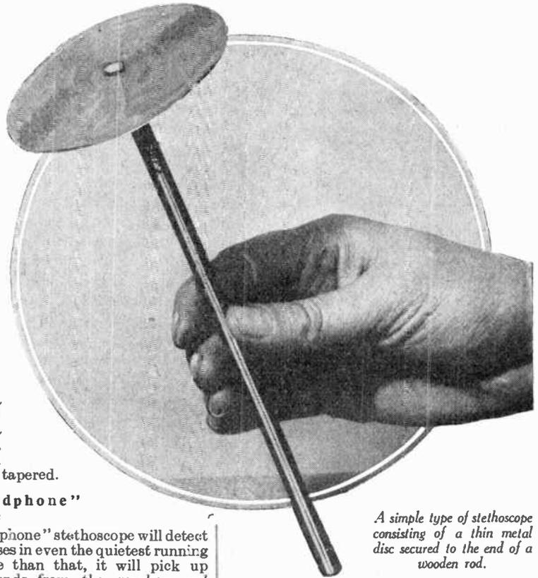
A simple type of stethoscope consisting of a thin metal disc secured to the end of a wooden rod.
