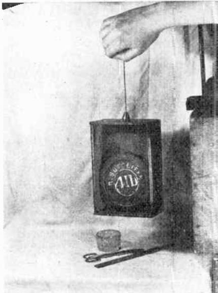
A wooden box containing a 4-lb. weight suspended by a liquid air-cooled piece of frozen metal to its outer side.
