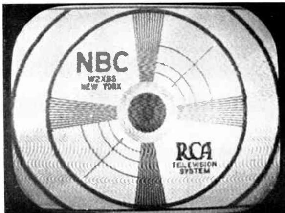
Figure 45—Excessive Diathermy Interference
