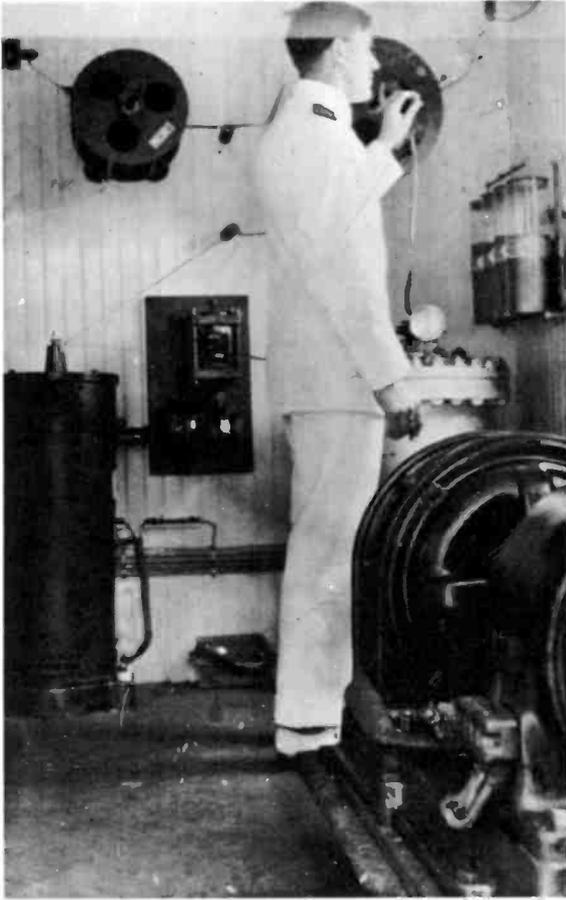
*Fred Muller, Chief Wireless Operator, S. S. Pastores, United Fruit Co. tuning up a 2-kw Fessenden Synchronous Nesco QS transmitter, in 1913. Note the 400-lb. compressed air condenser in background.*
