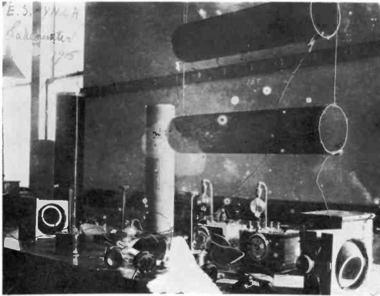
*Amateur station of the East Side Y.M.C.A. East 86th. St., New York City in 1915. The apparatus was installed and operated by Harry Sadewater who also gave a course of instruction in Wireless Telegraphy there. Note the long wave tuning coils and the two variometers and Audion bulbs.*
