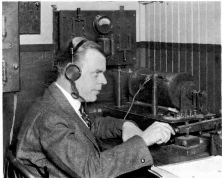
Jack Binns at the key of a reconstructed transmitter similar to the one with which he sent the first radio distress call (CQD) in history, from the sinking S.S. Republic in 1909.
