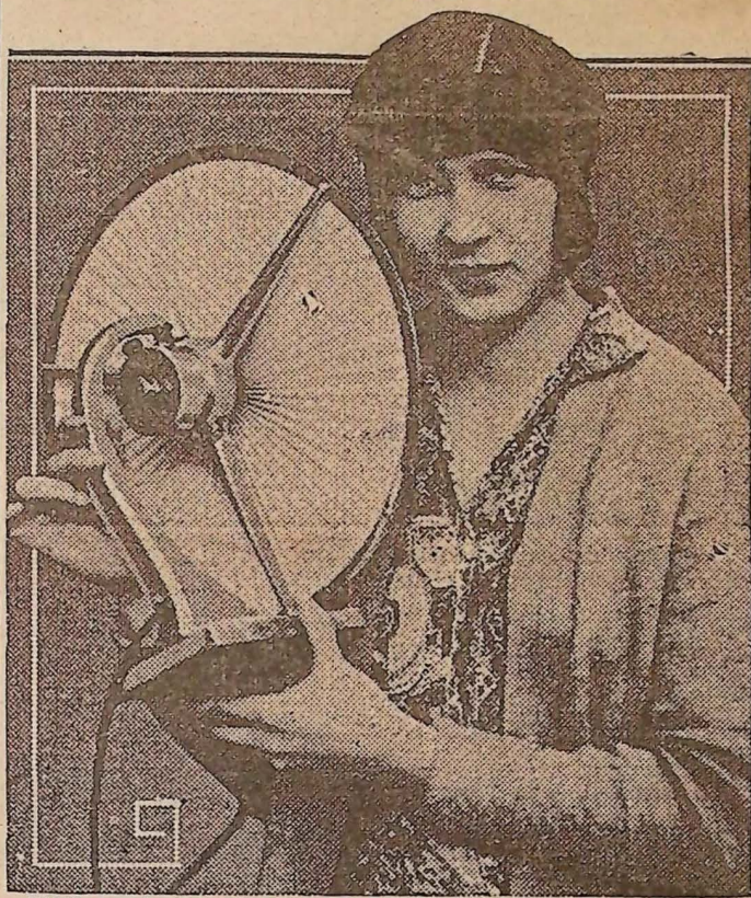
While you're combing your hair, or primping up, listen-in on a broadcasting station through this form of loud speaker. Miss Betty Pearce of Forest Hills, L. I., is shown with it. It's an accordion-pleated paper cone, instead of the horn type. It was invented by a French engineer.
