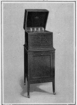
THE Radiola Grand has been especially designed to receive broadcasting stations operating on the standard wavelengths of 360 and 400 meters but an additional range is available up to 550 meters. The finest principles
