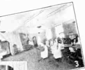
3.—The ensemble studio will accommodate a large orchestra or group of singers. It is draped with Monk's cloth and the ceiling is especially constructed to be acoustically efficient.
