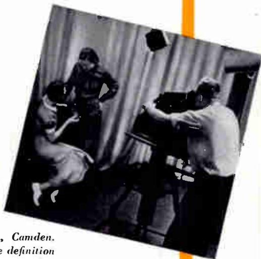
*Experimenting in the RCA Laboratories, Camden, N. J., in 1934. Such tests resulted in picture definition of 343 lines, a frame speed of 30 per second and a greatly improved synchronizing device.*
