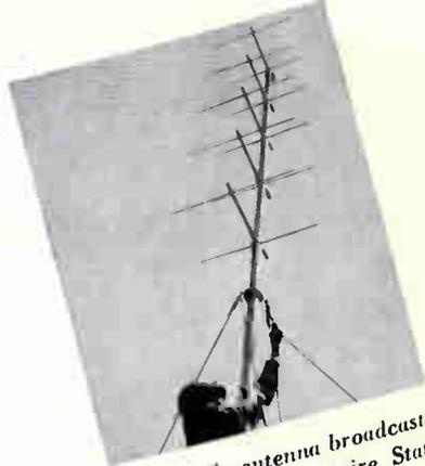
Telemobile antenna broadcasts field pickup to Empire State transmitter for re-broadcast.
