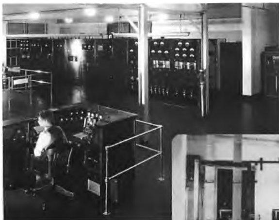
Figure 73. (Left) Another view of the Western Electric 7A 50-kW transmitter used as the exciter for the 500-kW transmitter. Engineer Dick Walker is seated at the console which controlled the operation of both transmitters, 1934.
