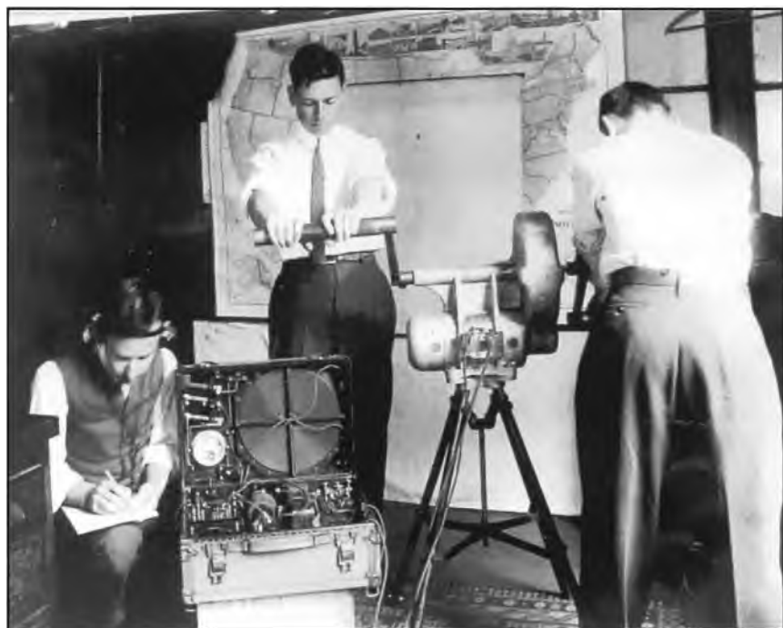
Three men demonstrate the operation of a pack set with a hand generator. The photograph, probably dating to 1916, is from the Radioana Collection, Archives Center, National Museum of American History, Smithsonian Institute. This is one of the many rare photographs which trace the evolution of wireless pack sets in the article in this issue by Russ Kleinman and his coauthors.
