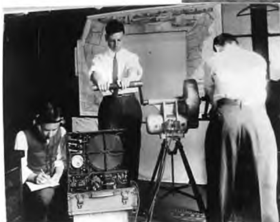
Figure 3. (Left) Three men demonstrate the operation of a pack set with a hand generator. Probably about 1916.
