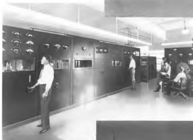
Figure 44. Western Electric Model 7A 50-kW transmitter at Mason, 1928.
