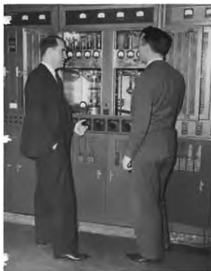
Figure 125. George Frederick (Fritz) Leydorf, Radiation Engineer and Floyd Lantzer, Chief Engineer, standing in front of the 75-kW shortwave transmitter used for Crosley radio station WLWO. This transmitter was located in the WLW transmitter building near Mason, Ohio.
