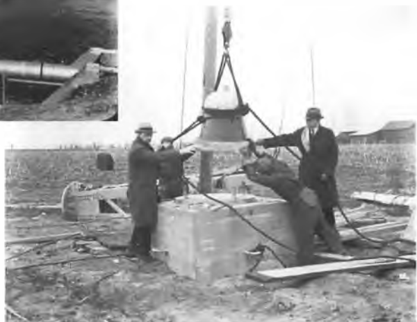
Figure 56. (Right) Bottom half of the antenna base insulator which supported the vertical antenna.
