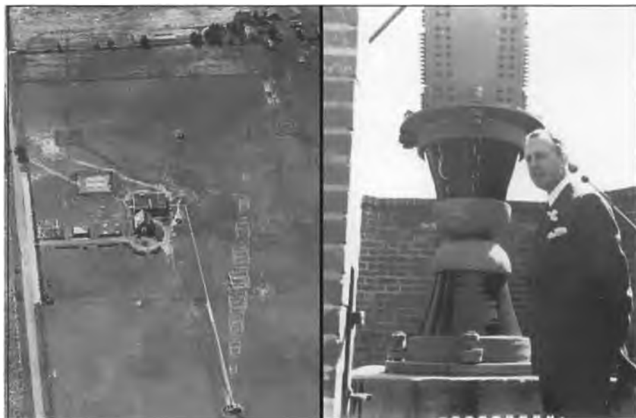
Figure 62. (Left) Aerial view of station WLW showing the vertical and the "T" antennas. Figure 63. (Right) Powel Crosley Jr. at the tower base insulator.
