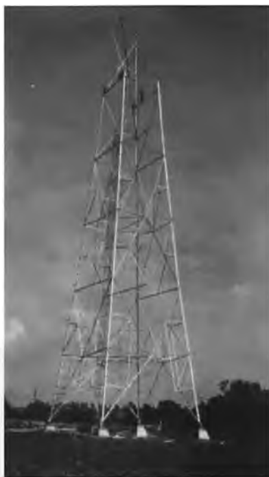
Figure 42. (Above) 300 foot self-supporting tower under construction.
