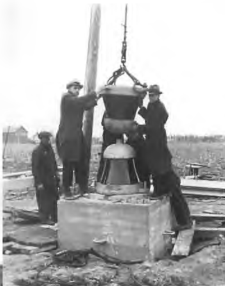
Figure 57. (Right) Top half of the base insulator which supported the vertical antenna.
