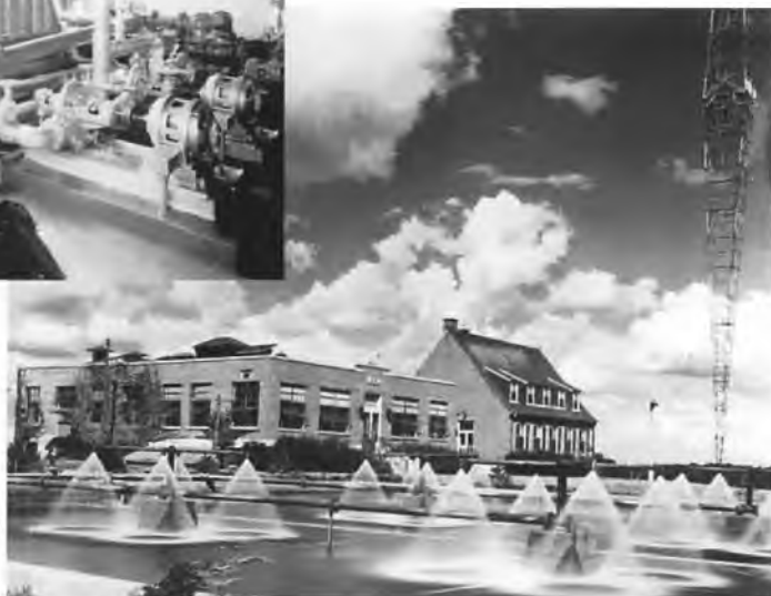
Figure 76. (Right) Heated water from the 500-kW transmitter was pumped to the outdoor spray pond to cool the 862 tubes, 1934.
