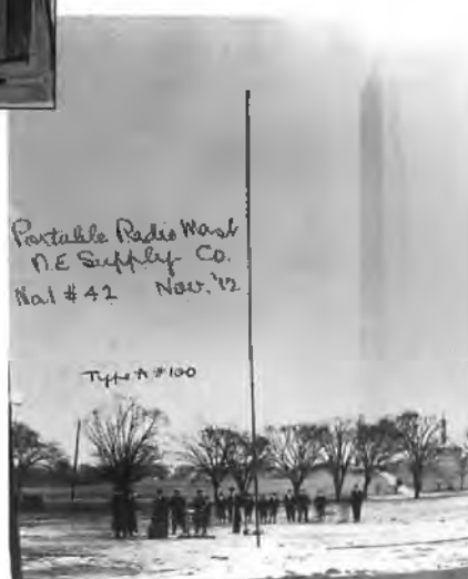
Figure 14. (Right) Standard Portable Aerial set up in front of Washington Memorial, in use with Type A pack set (serial number 100) made for the USN by N.E. Supply Co., 1912.
