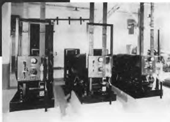
Figure 73. (Left) Another view of the Western Electric 7A 50-kW transmitter used as the exciter for the 500-kW transmitter. Engineer Dick Walker is seated at the console which controlled the operation of both transmitters, 1934.
