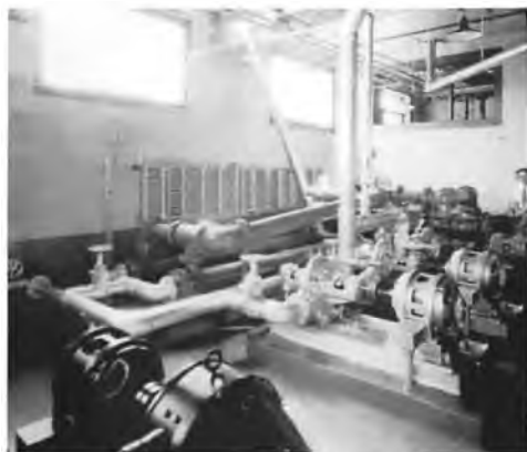
Figure 75. (Left) The pumps and heat exchangers for the 500-kW transmitter were located in the basement of the transmitter building and used to cool the 862 tubes, 1934.
