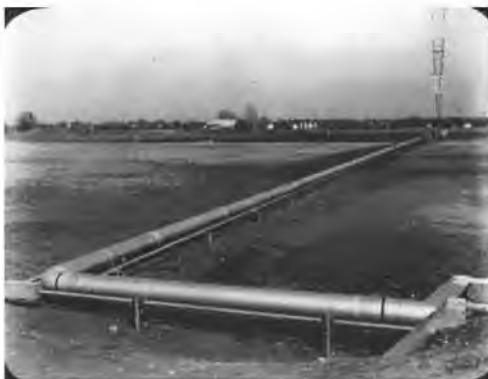
Figure 55. (Left) 100-Ohm coaxial transmission line to vertical antenna.
