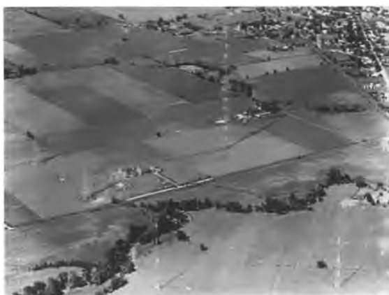
Figure 92. The WLW suppressor towers in the foreground provided directivity and reduced the signal strength in areas where interference was a problem, 1934.
