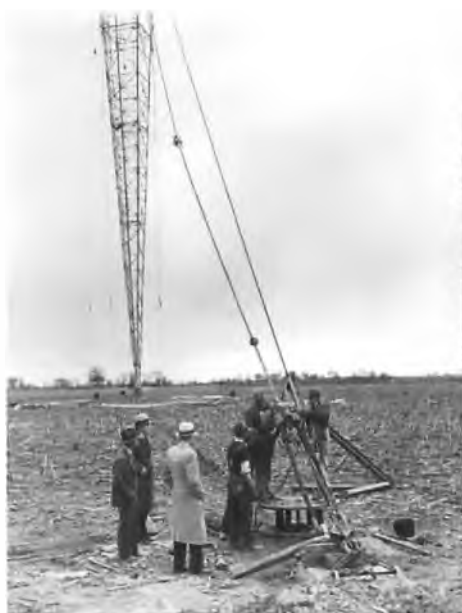
Figure 58. (Left) Guy cable installation used to support the vertical antenna.
