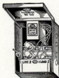
FIG. 115. Tobe Filterette 110. This Filterette is approved by Underwriters Laboratories for installation in any 110-volt circuit carrying 5 amperes or less.
