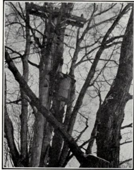
FIG. 87. Careful trimming of trees is required to avoid tree grounds and consequent interference.
