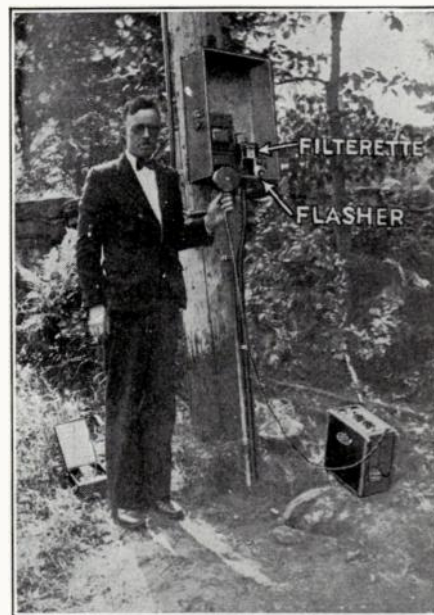
FIG. 65. Checking interference from a traffic flasher.
