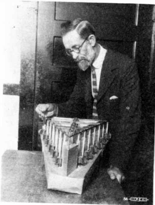
According to George E. Faucher, its inventor, a pier constructed like the model shown above will furnish an entire city with its electricity. The first model was exhibited in Los Angeles. Built like a pier 1,000 feet long, the "V" of the machine points oceanward and as the waves roll in they are split and operate two series of turbines on each side. The turbines are of steel and encased in air- and water-tight tanks that float.
