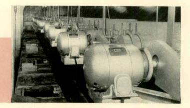
for a tremendous number of compressor, pump, and fan motors. Many of these had to be highly specialized types since they operate in the atmosphere of a refrigerant such as freon.
