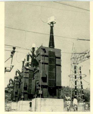
Here data is being obtained for construction of lines above the 287-kv limit. Shown are the 500-kv transformers and lightning arrester on the experimental lines at Tidd station.
