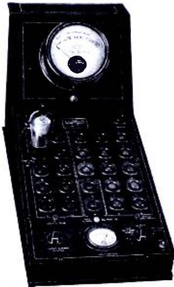
The Radio Products Co., Dayton, Ohio, have recently placed on the market their type 360 display tube tester, with large meter calibrated in layman's language. This meter mainly designates whether a tube is good or bad. The manufacturers of this tube tester state that the set owner does not understand the technical terms which are applied to radio tubes, but he is interested in knowing whether his tubes are good or bad.
