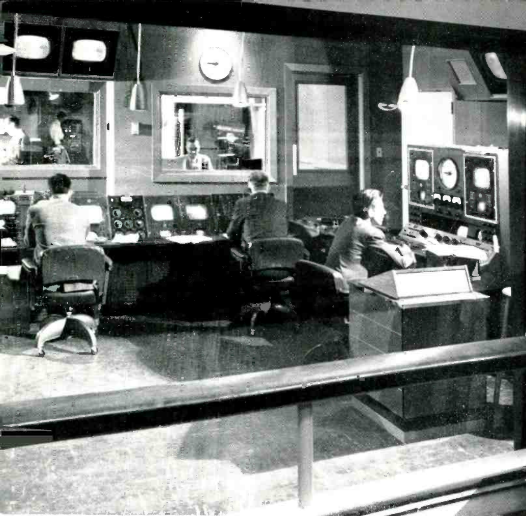
FIG. 1. This is the WCAU TV Master Control Room as seen through the window from the main lobby. The film and announce camera monitoring positions are at the long console on the far side of the room. The master control switching console, especially built by RCA to WCAU's specifications is at the extreme right. Part of the projection room can be seen through the window at the left. The window further right looks into the announce booth, and through a second window into the part of the projection room where the announce cameras are located.
