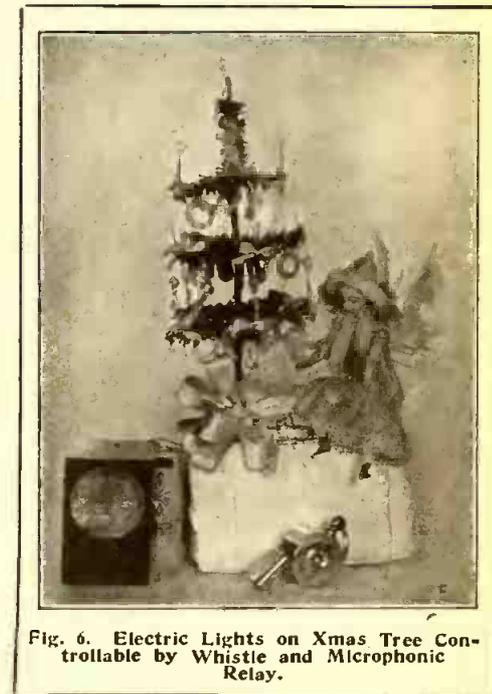
Fig. 6. Electric Lights on Xmas Tree Controllable by Whistle and Microphonic Relay.
