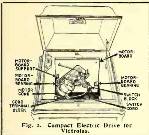
Fig. 2. Compact Electric Drive for Victrolas.
