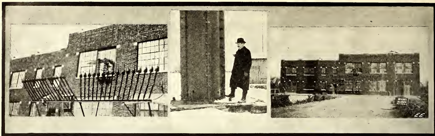
View at Left—A Close-up of the Thirty-two Wire Antenna Lead-in Entering the New Brunswick Station. Center—Mr. Alexanderson Standing at the Base of One of the 400 Foot Aerial Masts. Right—General View of Antenna Side of New Brunswick Trans-Atlantic Radio Station, Thru Which Station Secretary Daniels Talked by Wireless Telephone to Europe.
